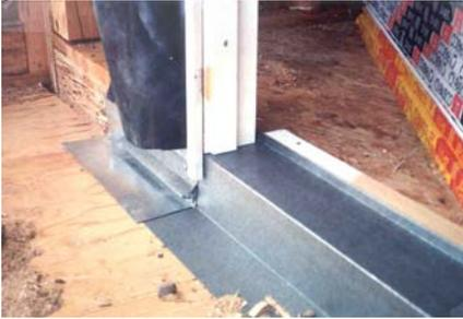
*This is an example of a sheet metal door pan. Code requires all terminations and doors be flashed properly.*
