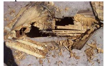
*Dry-rotted substrate needs to be replaced before new decking can be installed.*
