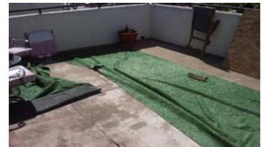
*Indoor/outdoor carpeting is bad for decks, they trap water underneath!*
