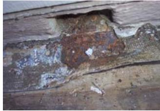
*Rusted metal is revealed after old coating was removed. This scupper must be replaced to properly waterproof the deck.*
